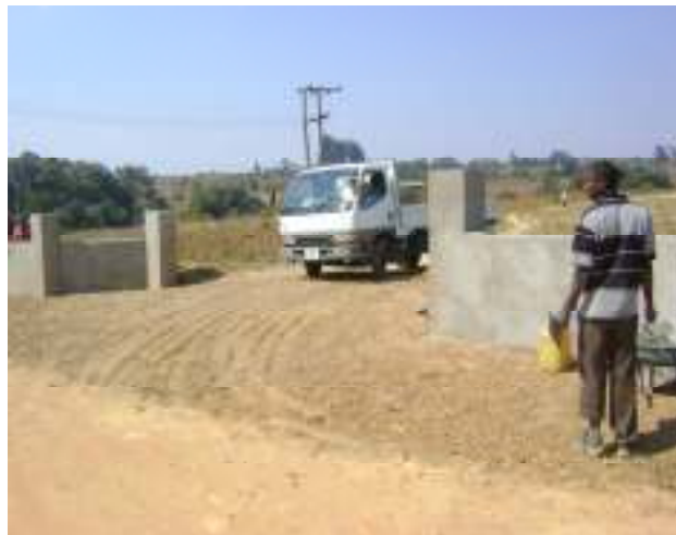
Gate way well designed to include guard's Shelter in future.
