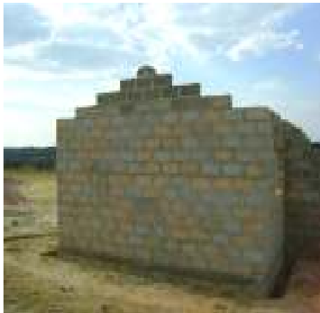
About to finish building
