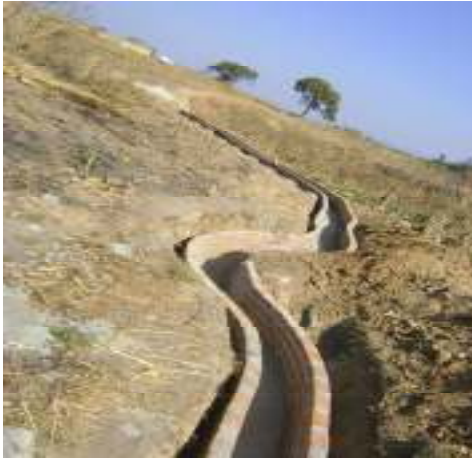
furrow construction in progress
