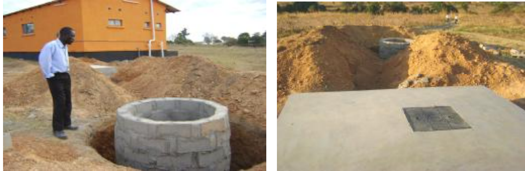
Sewer System still under Construction
